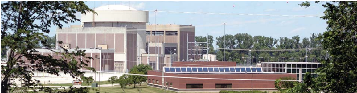
Fort Calhoun Station
