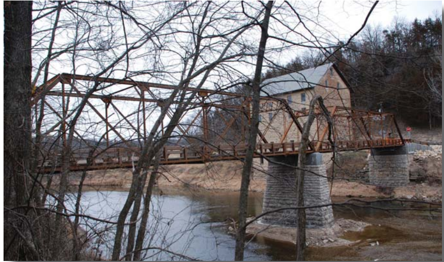
New Motor Bridge completed in November 2012.
