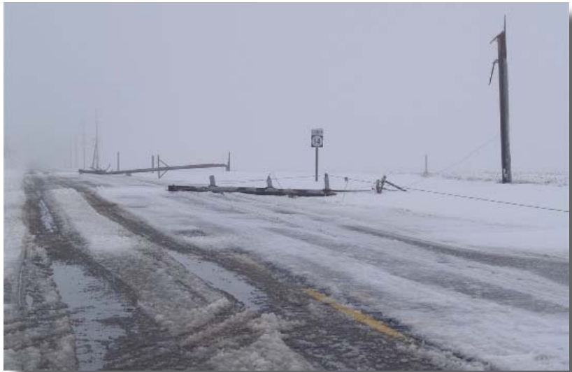
Downed power lines during a winter storm in Iowa.
