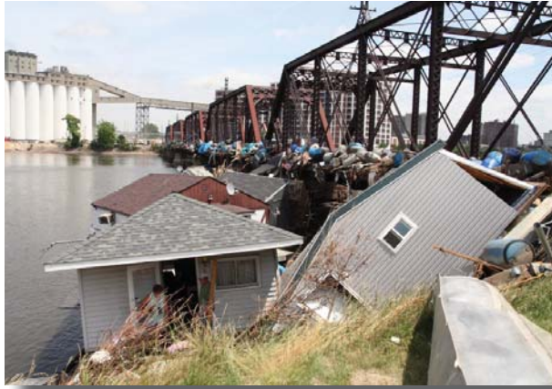
Union Pacific Railroad Bridge in Cedar Rapids, June 2008. FEMA photo.
