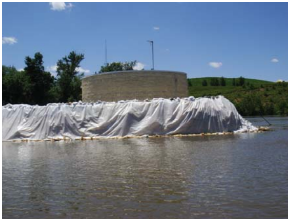
Sandbagging around the Iowa City Well House during June 2008 flooding. Photo by HSEMD.
