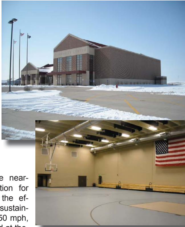
Palo's Community Center Tornado Safe Room. Photos by Kurt Hoffman, HSEMD.
