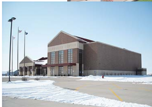
Left: The outside of the Palo Community Center safe room, constructed with Hazard Mitigation Program funds.
