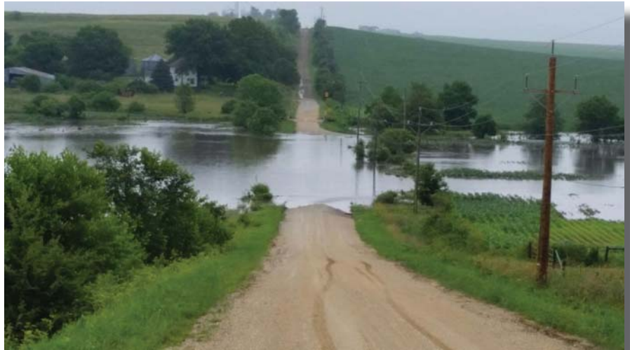
June 2015 flooding of Middle River near the town of Casey.
